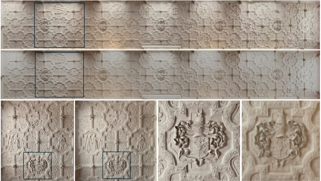
Figure 11: Comparisons of 3DGS (top, left) and MVS+Poisson Meshing (bottom, right) reconstruction of the whole ceiling in low-LOD.
